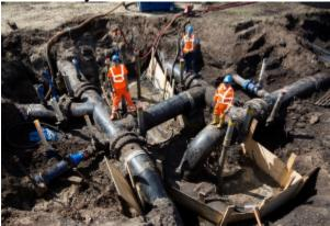
Subsidence can cause gas and water pipelines to break right where they enter houses. In the Netherlands, satellite data are used to monitor gas pipelines at affordable costs.
