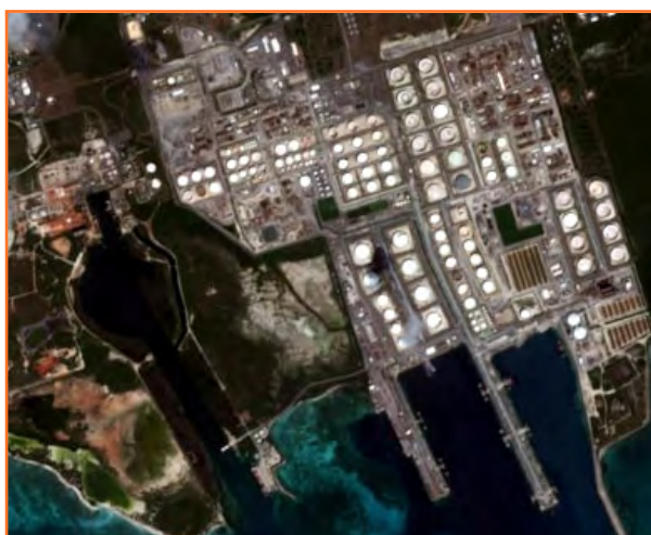
Figure 1: An oil storage facility including cylindrical storage tanks. (copyright Kayros)
