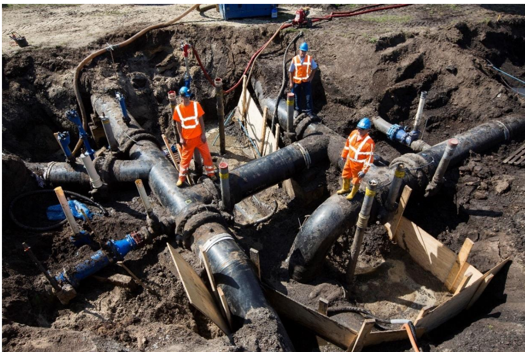
Figure 2-7: Water pipe maintenance (courtesy of Oasen).
