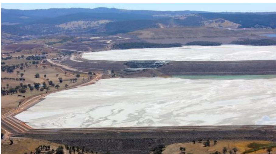
Figure 3-11: Cadia gold mine, Australia, tailings dam collapse.
