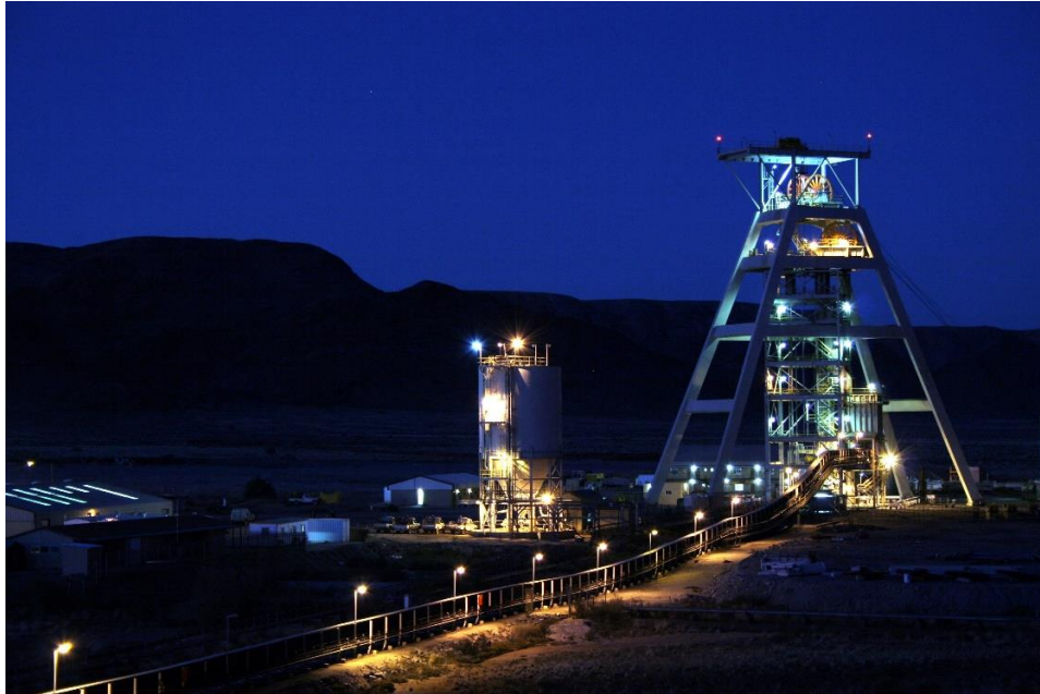
Figure 11 – Mine Shaft in South Africa
