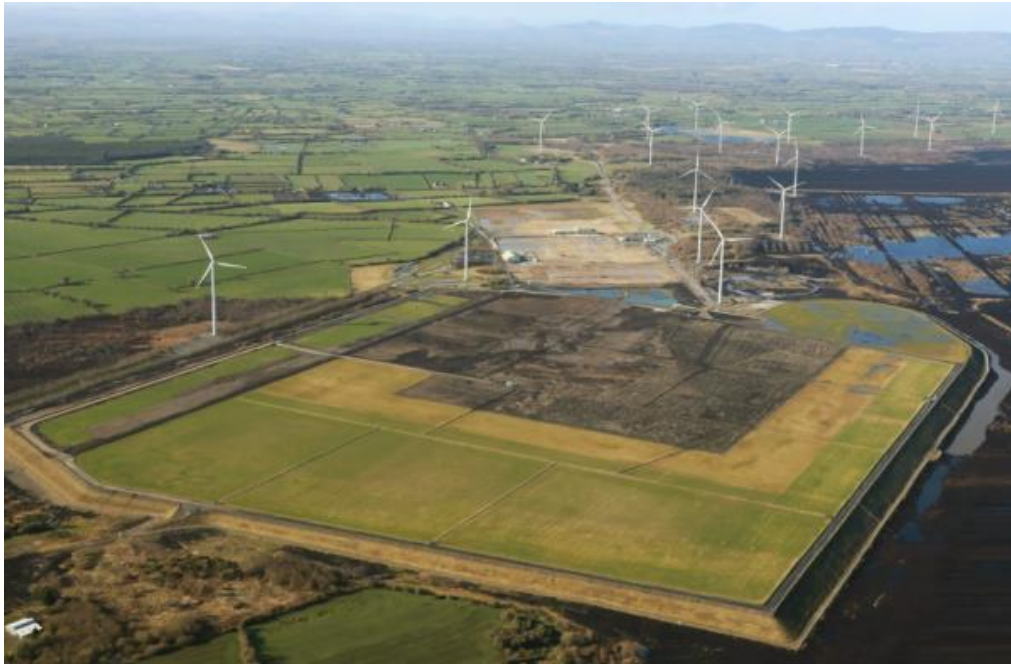
Figure 27 – Lisheen Mine – Tailings Management Facility 2018 – Rehabilitation almost complete
